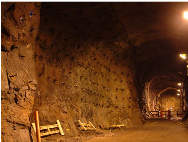
The shallow niche NASQ0036A in the TASQ-tunnel
